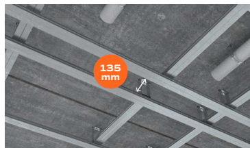
Installation width between profiles: 135 mm / ≈ 5,31".
