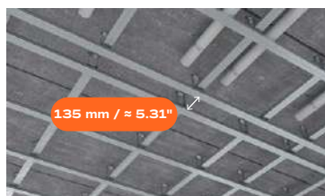
Installation width between profiles: 135 mm / \approx 5.31"
